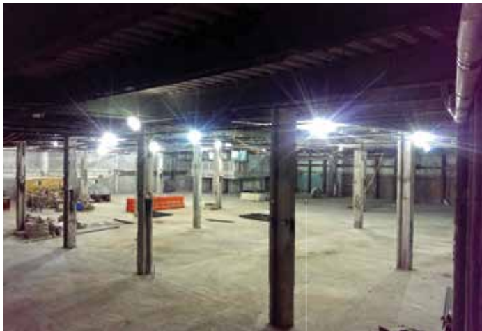
Figure 5. New double story space with reinforced columns.
