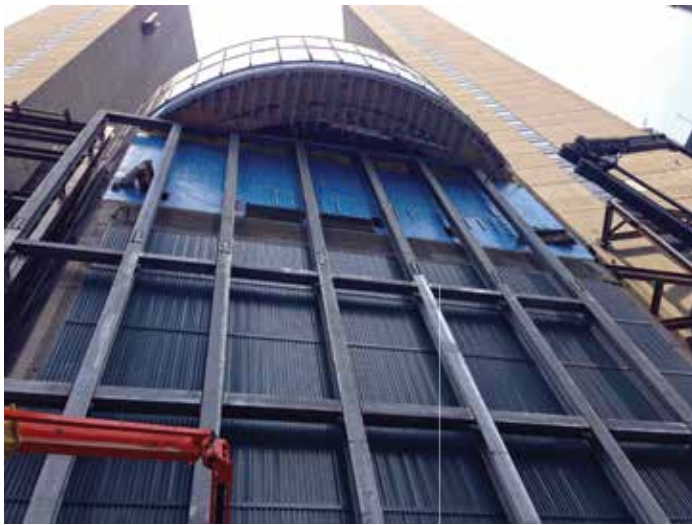
Figure 3. Vierendeel truss.
