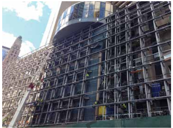
Figure 4. Installation of LED sign.
