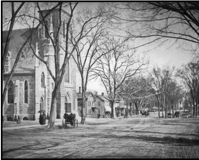
Main Street in 1875 - St. Peter's Church is on the left
