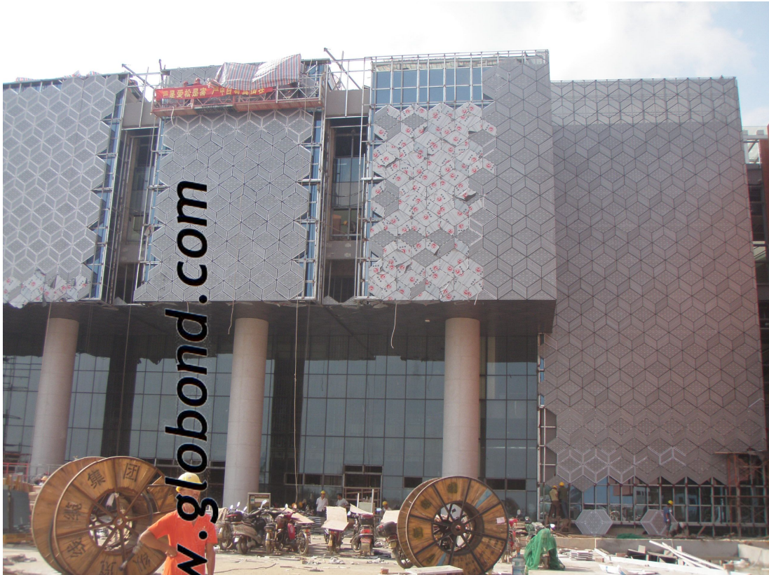
Perforated panels as curtain wall.
