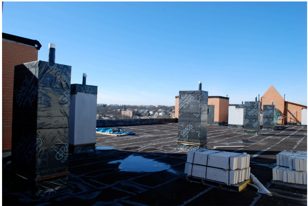
Roof – Acquisition Condition
