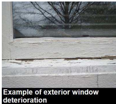
More window deterioration
