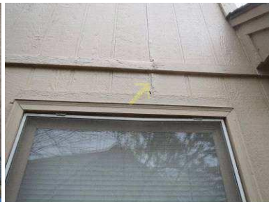
Siding/trim deterioration
