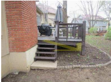
More than normal slant of deck
