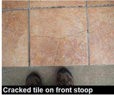
Cracked tile on front stoop
