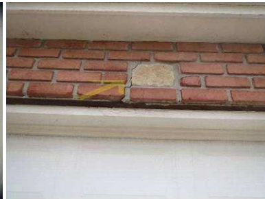
Crack around stone
