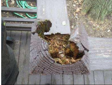
Rotting deck railing post
