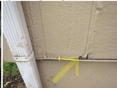
Siding/trim deterioration
