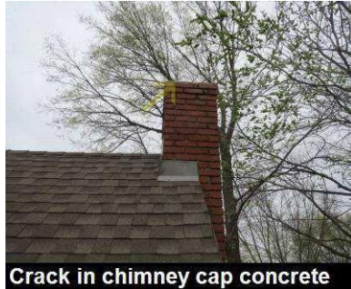
Crack in chimney cap concrete
