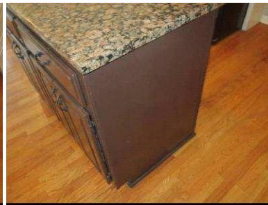
Should be an electrical outlet
