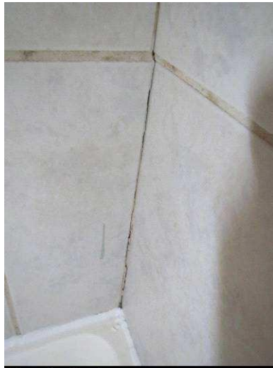
Grout missing
