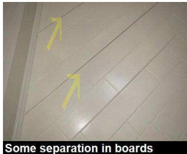
Some separation in boards
