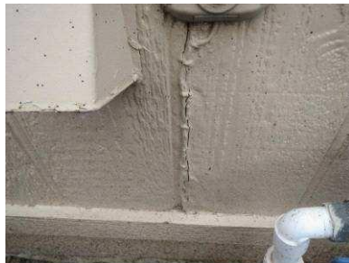
Siding/trim deterioration
