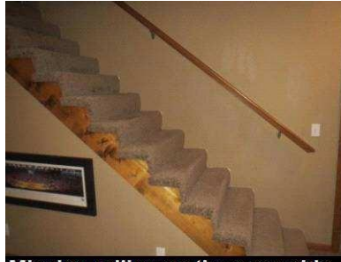
Missing railing on the open side of stairs
