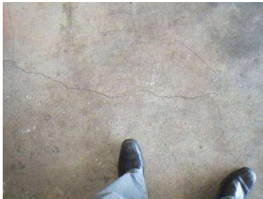
Minor cracks in garage floor
