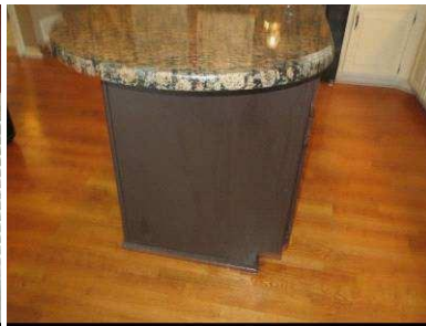
Should be an electrical outlet
