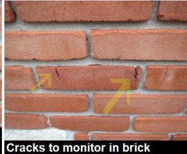
Cracks to monitor in brick
