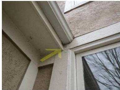
Siding/trim deterioration
