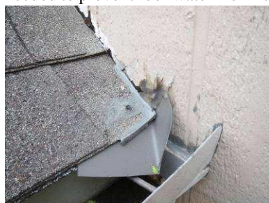
Attempted flashing kickout installation
