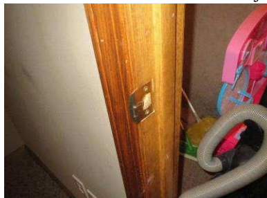
Door does not latch-SE corner bsmt closet
