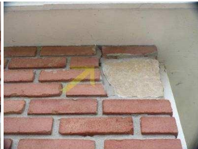
Crack around stone
