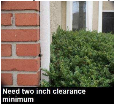
Need two inch clearance minimum
