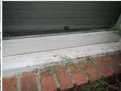
Siding/trim deterioration
