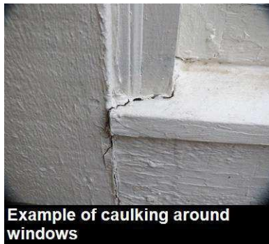
Example of caulking needed on siding seam
