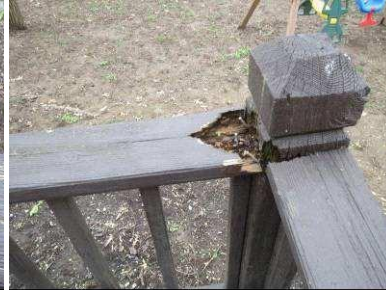
Rotting top railing
