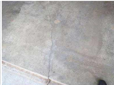
Minor cracks in garage floor
