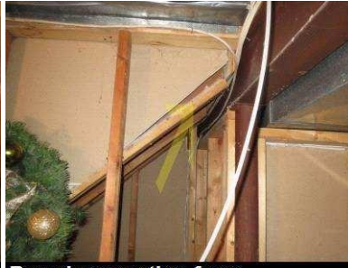
Board separating from structure
