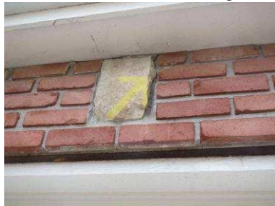
Crack around stone
