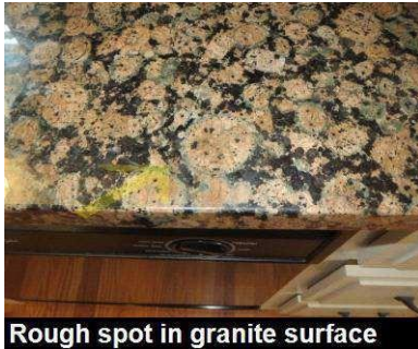
Rough spot in granite surface
