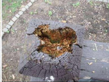
Rotting deck railing post
