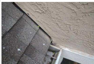
Needs flashing kickout installed
