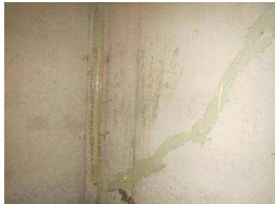
Basement wall repair work
