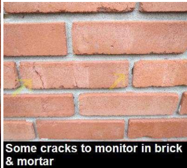
Cracks to monitor in brick
