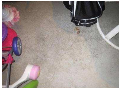
Minor floor cracks in basement
