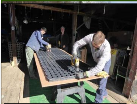
Assembling 12.7' geoblock sections
