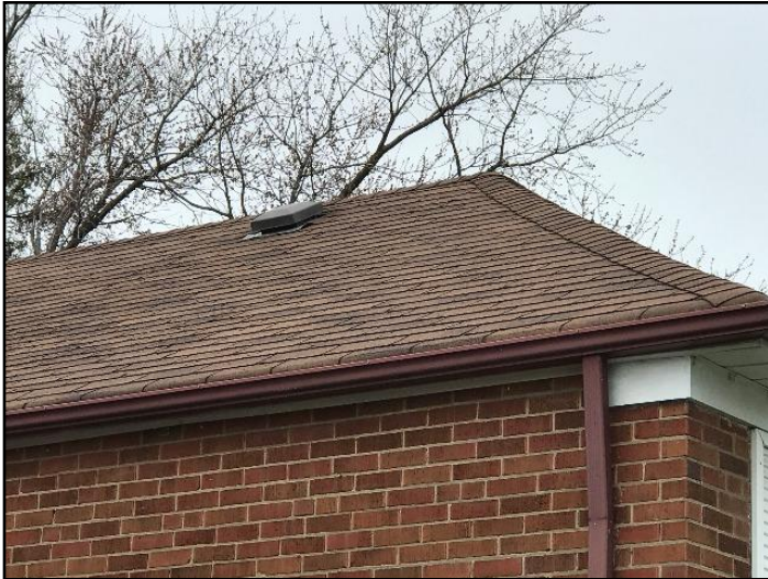
1. Asphalt shingles
