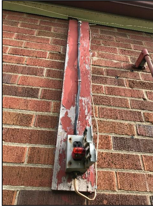
36. No GFCI/GFI (Ground Fault Circuit...
