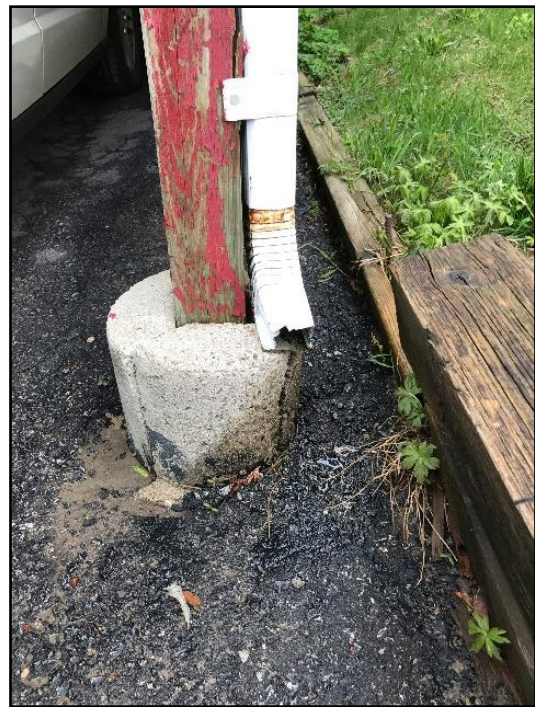
16. Should discharge 6 feet from building
