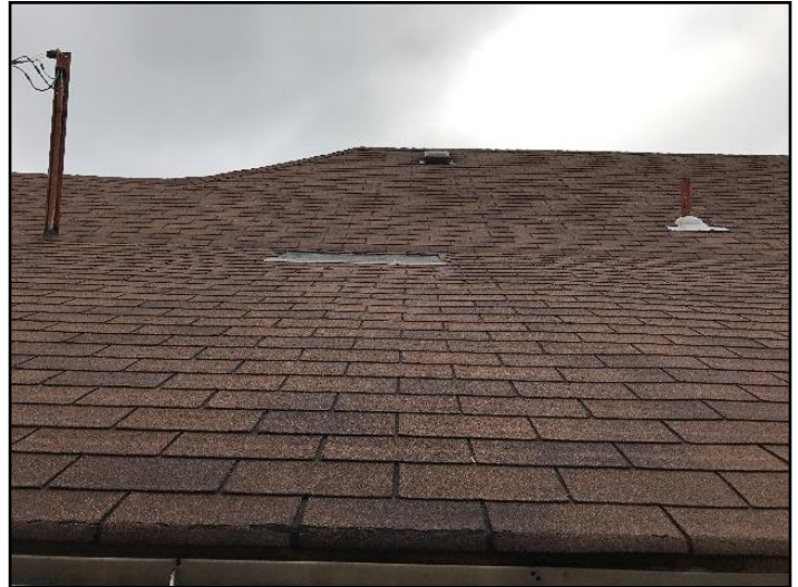
2. Asphalt shingles
