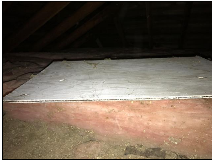
48. Not insulated and not weatherstripped
