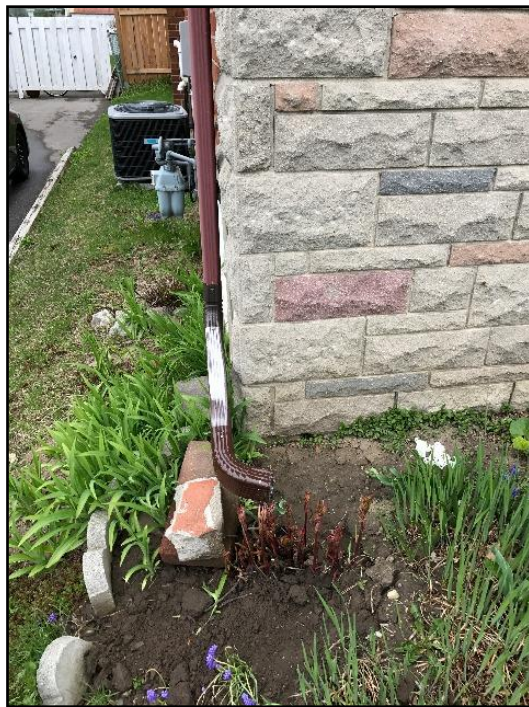
15. Should discharge 6 feet from building
