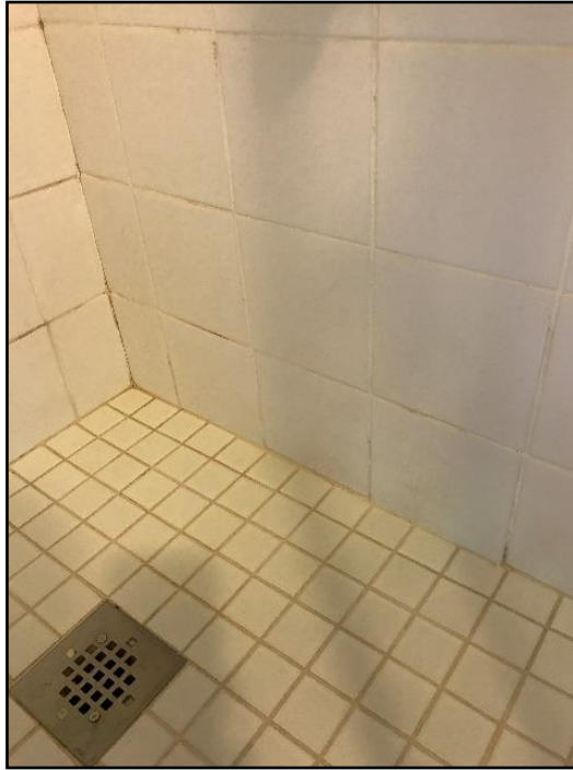
55. Caulking loose, missing or deteriorated
