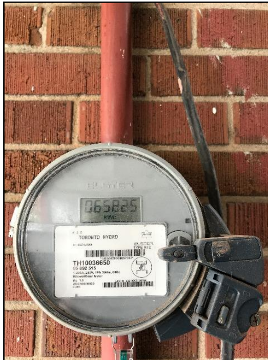
26. Meter is rated for 200 Amps
