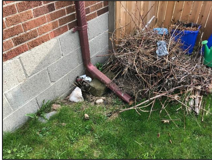
17. Should discharge 6 feet from building
