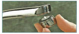
• Reassemble the aerator by screwing it back onto the faucet and hand-tighten.
