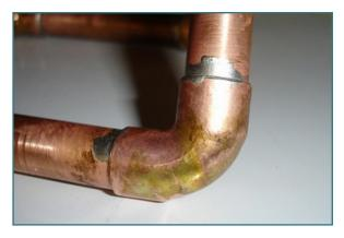
Copper pipes joined by lead solder.
