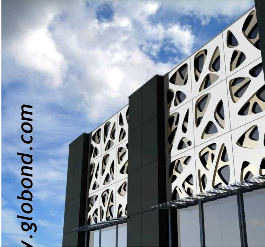
Aluminium panels engraved as cladding decoration .
