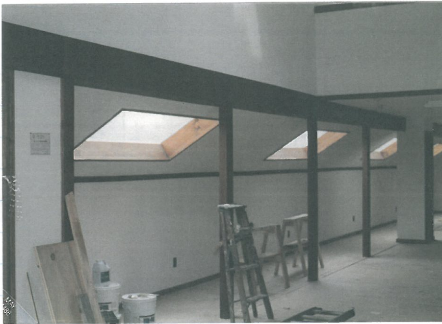
"skybox" under construction
