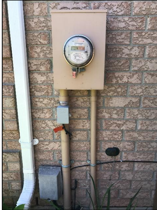
15. Underground - cable material not visible
