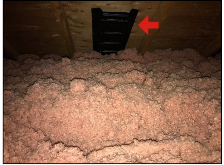
30. Soffit vent (view from the attic)
