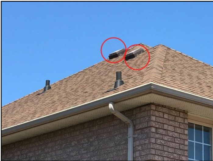
27. Roof vent (view from exterior)
