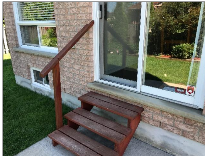
10. Spindles (balusters) missing
