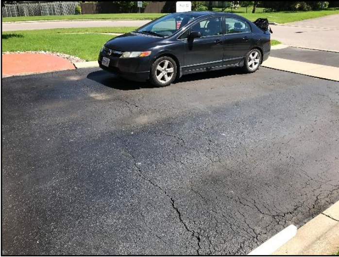
11. Cracked, settled, or damaged surfaces
