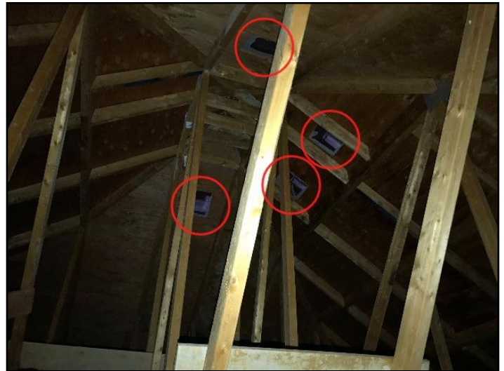
28. Roof vent (view from the attic)
