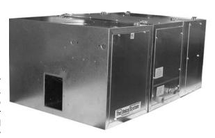
and plenums. Supply ducts to individual rooms are only 2-inch (50 mm) inside diameter, and can be run over or around structural obstacles or through existing walls and closets where conventional duct will not fit. Plenum duct inside dimensions are 7, 9, or 10-inch. Older buildings, custom homes, commercial offices, and other applications can be air conditioned and heated with a Unico System without major renovations or sacrifice of space.
